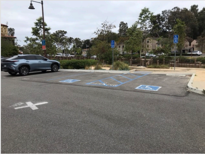
OVERVIEW OF ACCESSIBLE PARKING AREA
