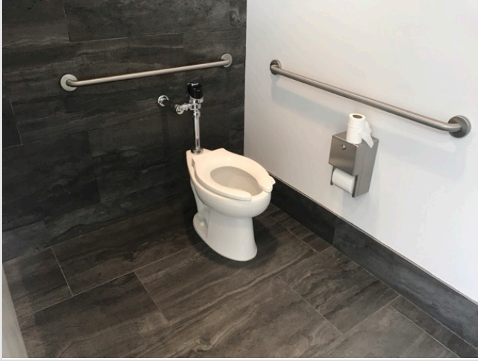
TOILET STALL OVERVIEW
