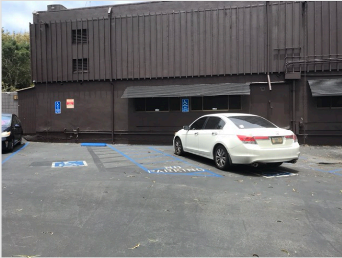
OVERVIEW OF ACCESSIBLE PARKING AREA
