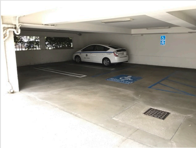
OVERVIEW OF ACCESSIBLE PARKING AREA
