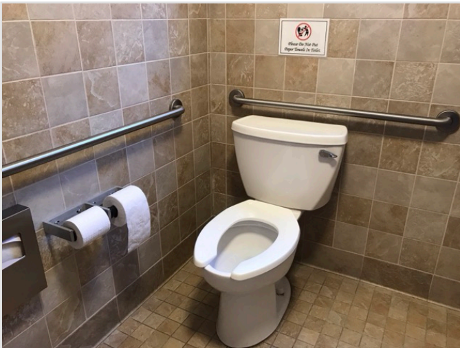
TOILET STALL OVERVIEW
