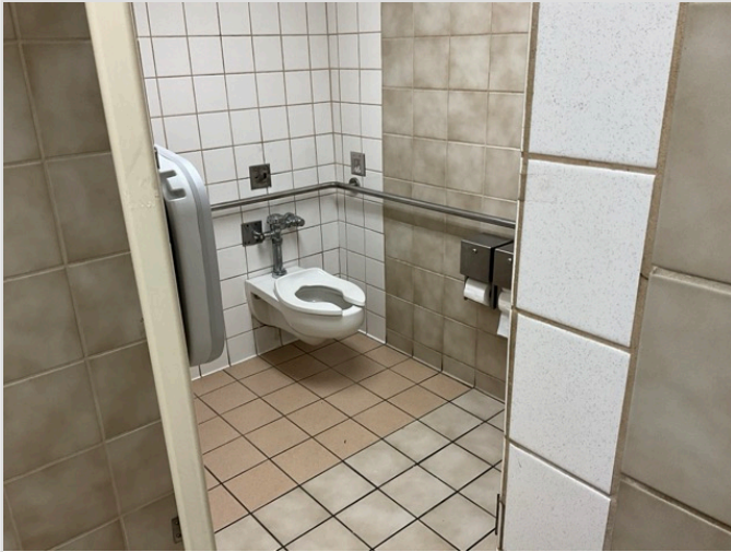
TOILET STALL OVERVIEW
