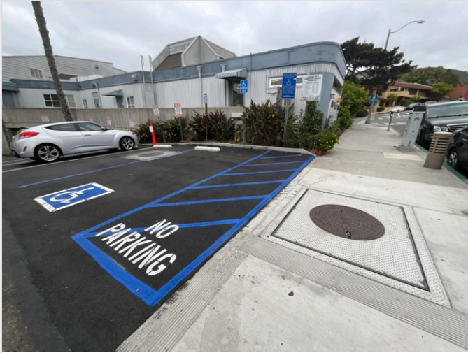
OVERVIEW OF ACCESSIBLE PARKING AREA
