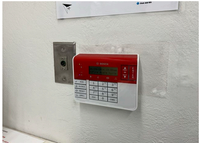
12 – FIRE ALARM / SECURITY
