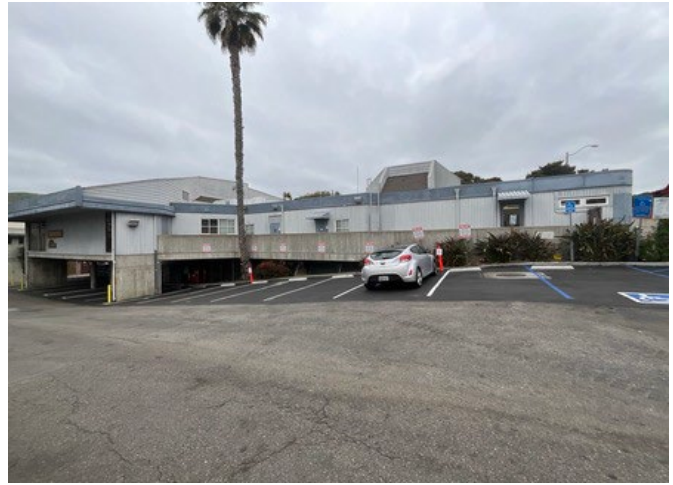
2 – PARKING LOTS OVERVIEW
