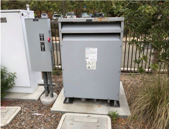
7 - SECONDARY TRANSFORMER
