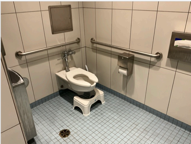
TOILET STALL OVERVIEW
