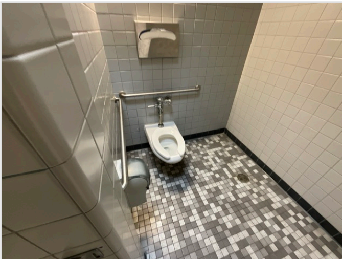
TOILET STALL OVERVIEW
