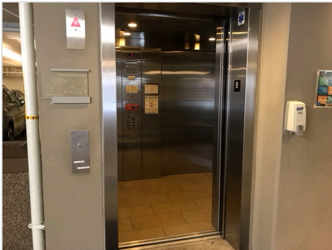
LOBBY LOOKING AT CABS (WITH DOORS OPEN)
