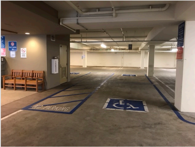
OVERVIEW OF ACCESSIBLE PARKING AREA
