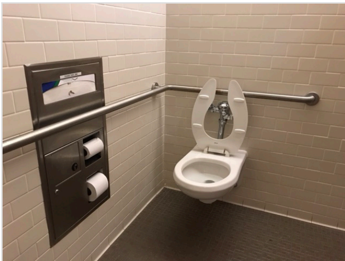
TOILET STALL OVERVIEW
