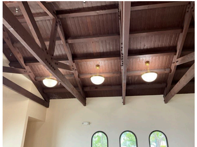
14 - INTERIOR LIGHTING SYSTEM
