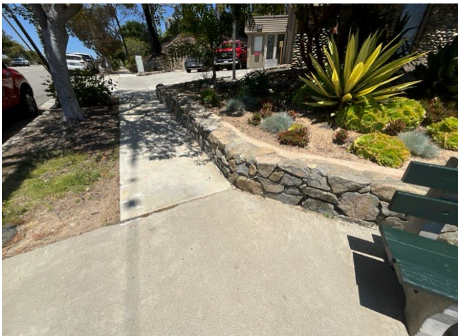
5 – RETAINING WALL AND WALKWAYS
