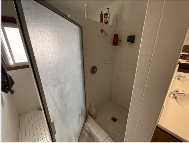
SHOWER NOT ACCESSIBLE
