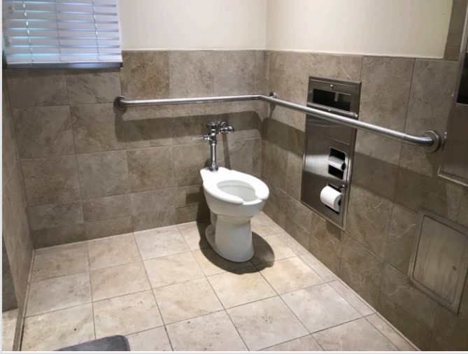
TOILET STALL OVERVIEW
