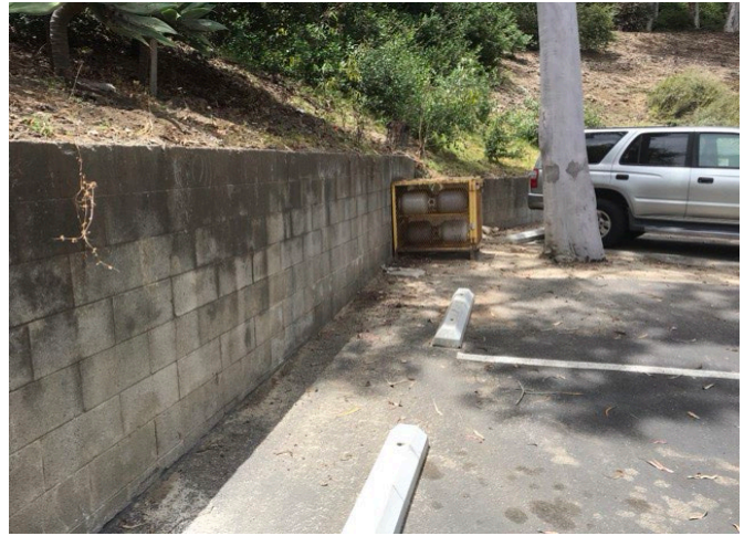
2 – CMU RETAINING WALL
