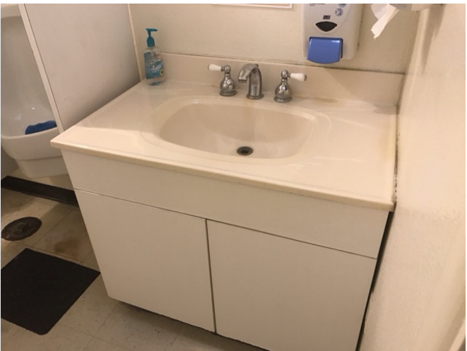
IRVINE BOWL BACKSTAGE LAVATORIES NO CLEARANCE/FAUCET HANDLES
