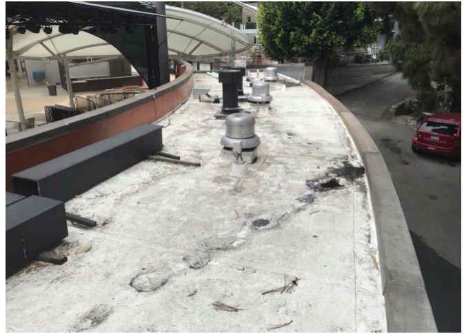
8 – ROOFING - GREEN STAGE BUILDING
