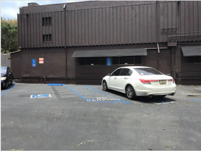
OVERVIEW OF ACCESSIBLE PARKING AREA
