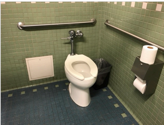
TOILET STALL OVERVIEW
