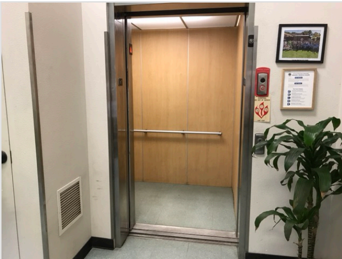
LOBBY LOOKING AT CABS
