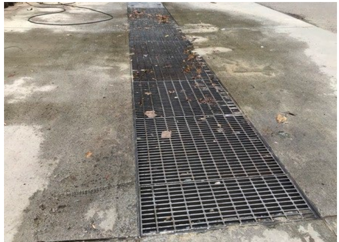
12 – DRAIN, SAND/GRAVEL INTERCEPTOR
