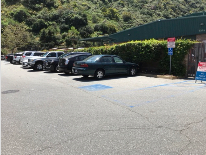
OVERVIEW OF ACCESSIBLE PARKING AREA
