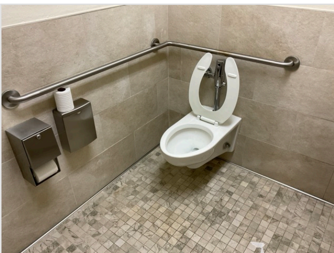
TOILET STALL OVERVIEW
