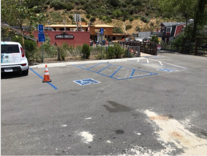
OVERVIEW OF ACCESSIBLE PARKING AREA
